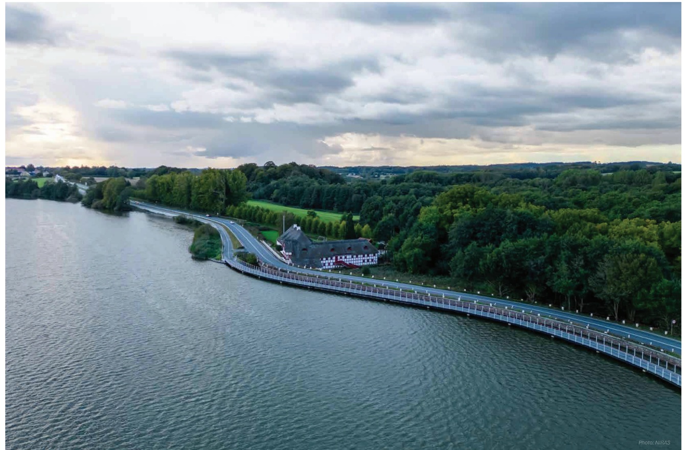
NIRAS supported Vejdirektoratet (The Danish Road Directorate) in establishing a 2.5-kilometre path for cyclists and pedestrians, which includes a bridge at Hvidkilde Lake. The bridge was constructed to enhance both comfort and safety for vulnerable road users on the old, narrow road.
